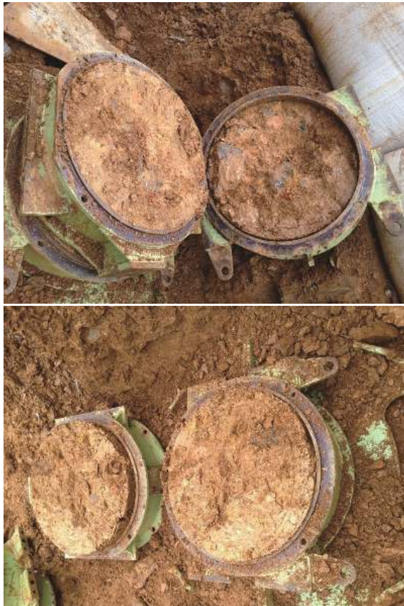
图 14 自反力双剪面大型剪切仪得到的典型剪切破坏面 Fig. 14 Shear failure interface attained through self-balanced in-situ shear equipment owning two shear interfaces
