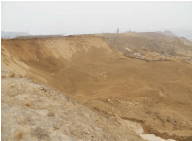
(a) 20150129陈家滑坡滑坡全貌
