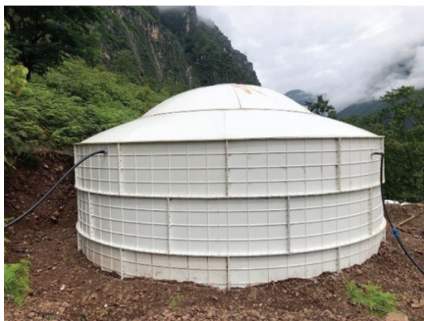
图7 昭觉县哈甘乡瓦西村地表—地下水联合调蓄示范工程 Fig.7 Demonstration project of surface-groundwater joint storage in Waxi Village, Hagan Town, Zhaojue County
