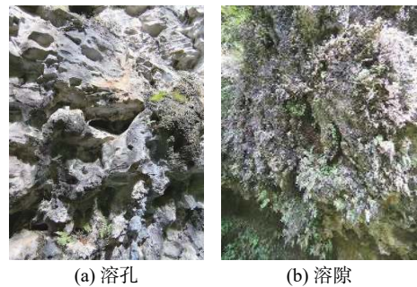
图 4 溶孔与溶隙 Fig. 4 Solution pore and solution gap
