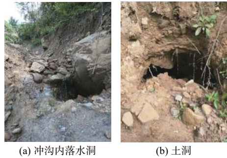
图 3 落水洞与土洞 Fig. 3 Water hole and soil hole
